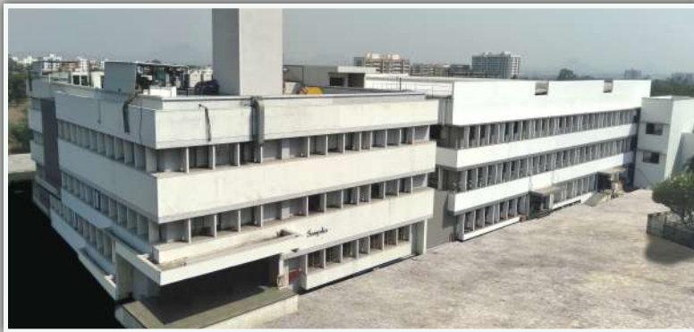
Rishabh Instruments HQ and Operational setup-Area- 10,240 Sq. Mtrs.
